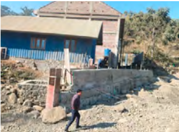
Retention Wall to Prevent further damage (Compassion)
