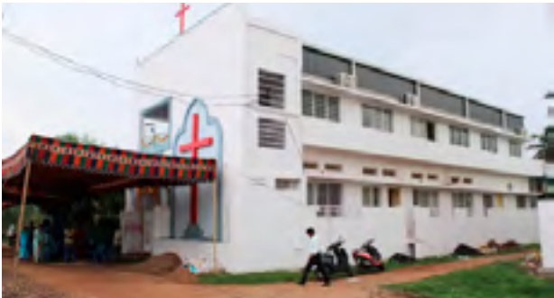
Church Renovation & Extension at Penamkuru (CREAM)
