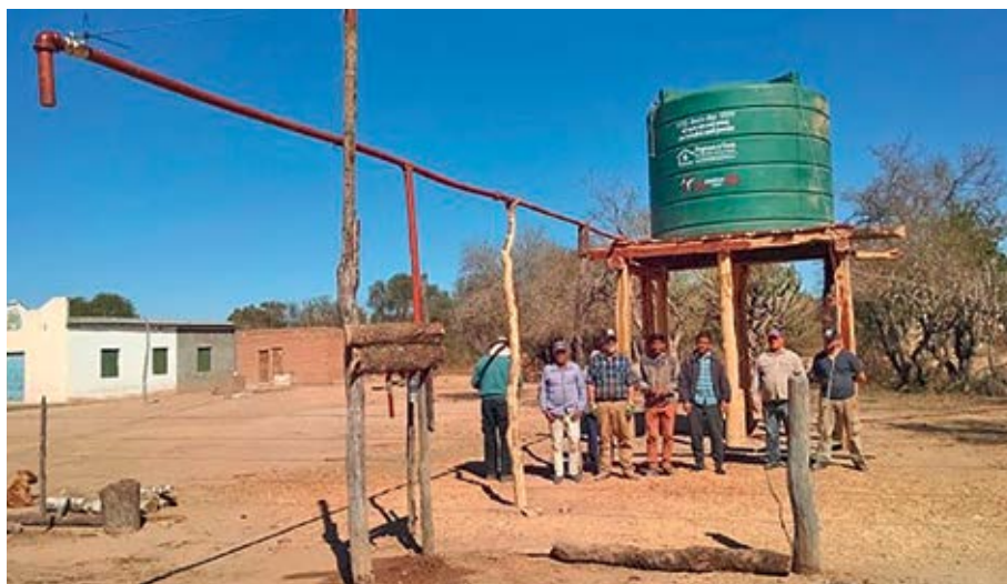
Water tank in Miraflores on a wooden structure
